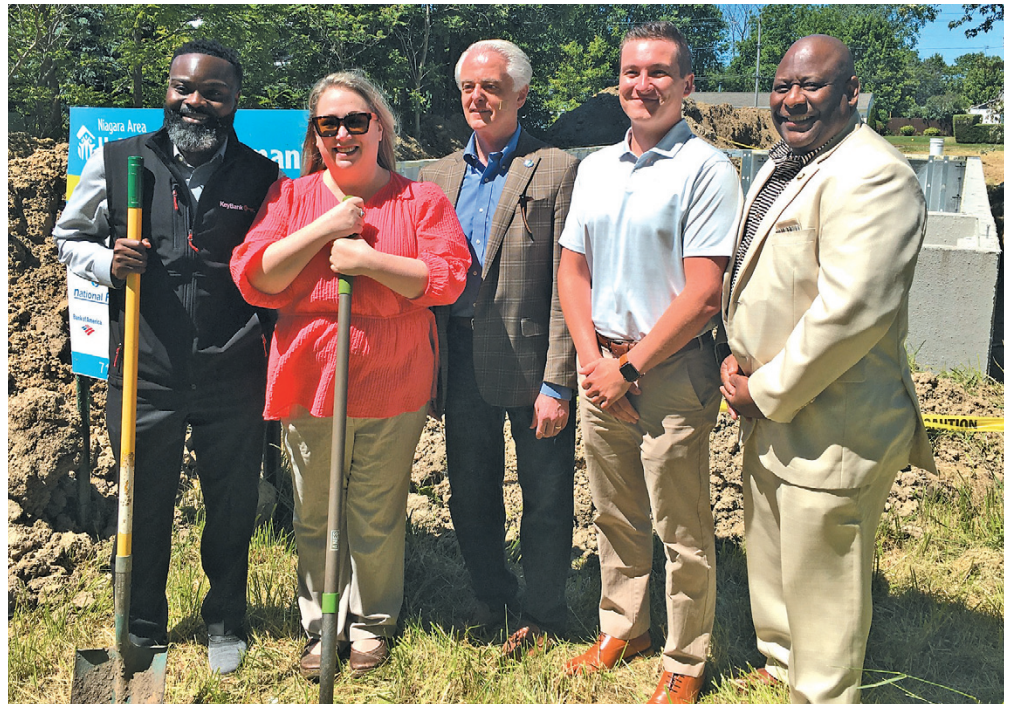
Habitat for Humanity celebrates the groundbreaking on their newest home in Niagara Falls. Pictured (left to right), Chiuwike Owunwanne of KeyBank, Habitat Executive Director Gina Beam, Niagara Falls Mayor Robert Restaino, Jeff Kwiatowski of National Fuel, and Fourth District Niagara County Legislator Jeffery Elder. (Submitted photo)
